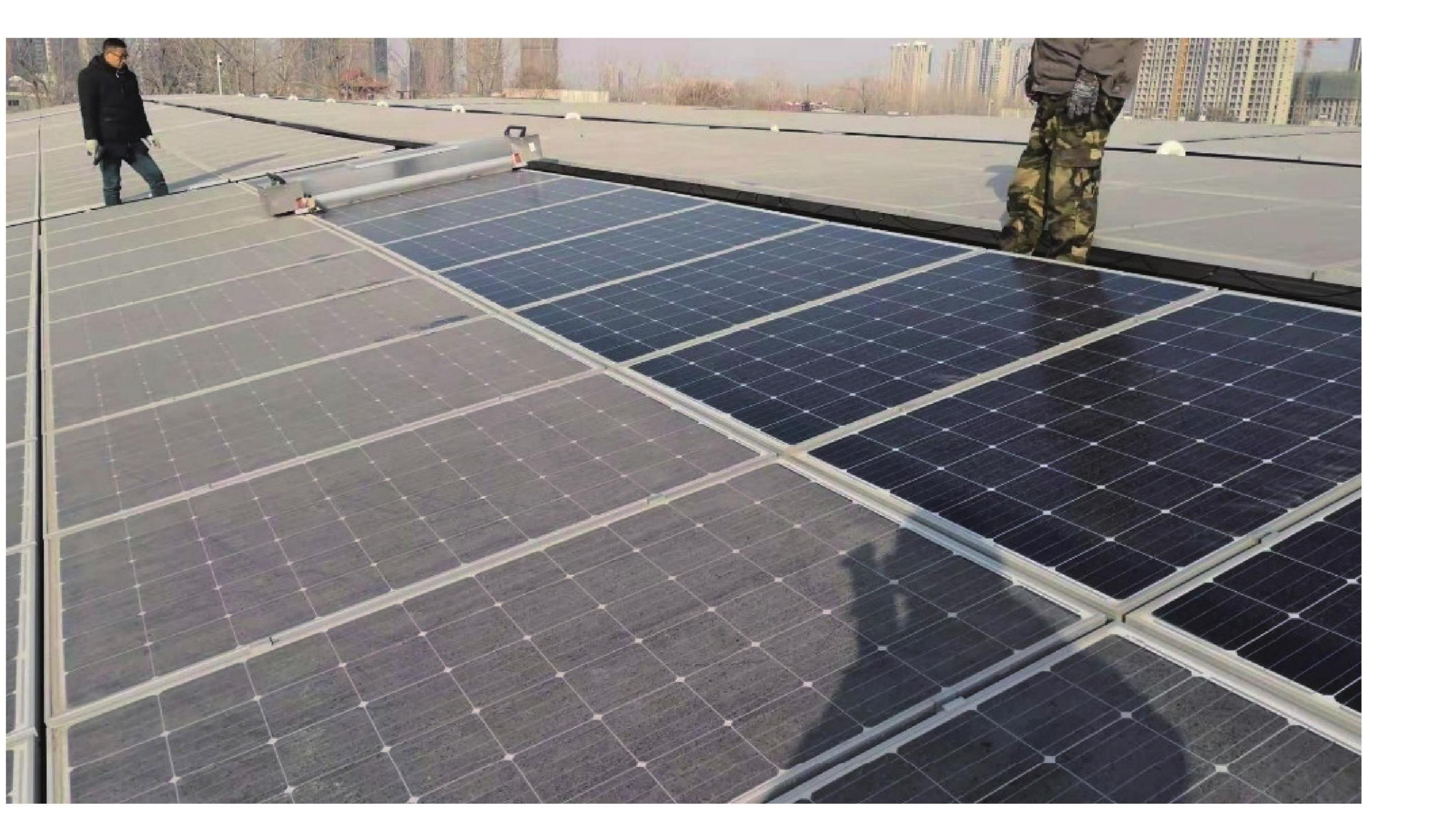
The solar panels covered by pollutant may cause hot spots, which will damage the panel and even make the panel burn.
