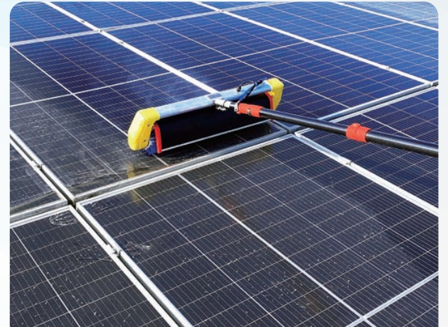
MULR-D Pro on factory rooftop system
